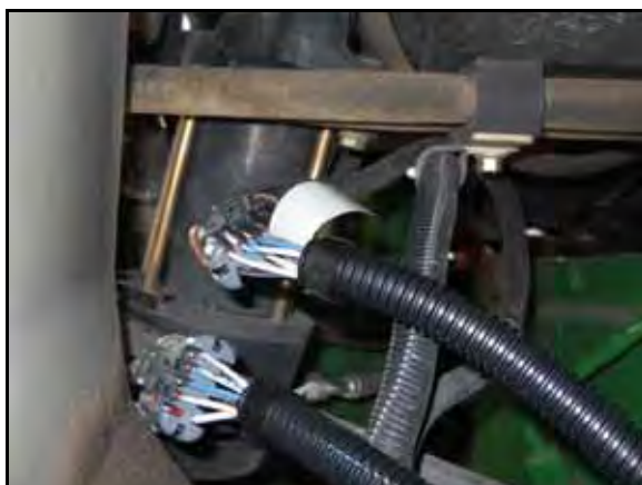
FIGURE 14. Valve Harness Connected to Steering Control Unit
