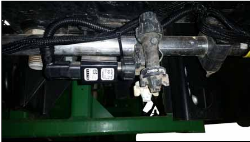
FIGURE 6. Securing Valve Branches
