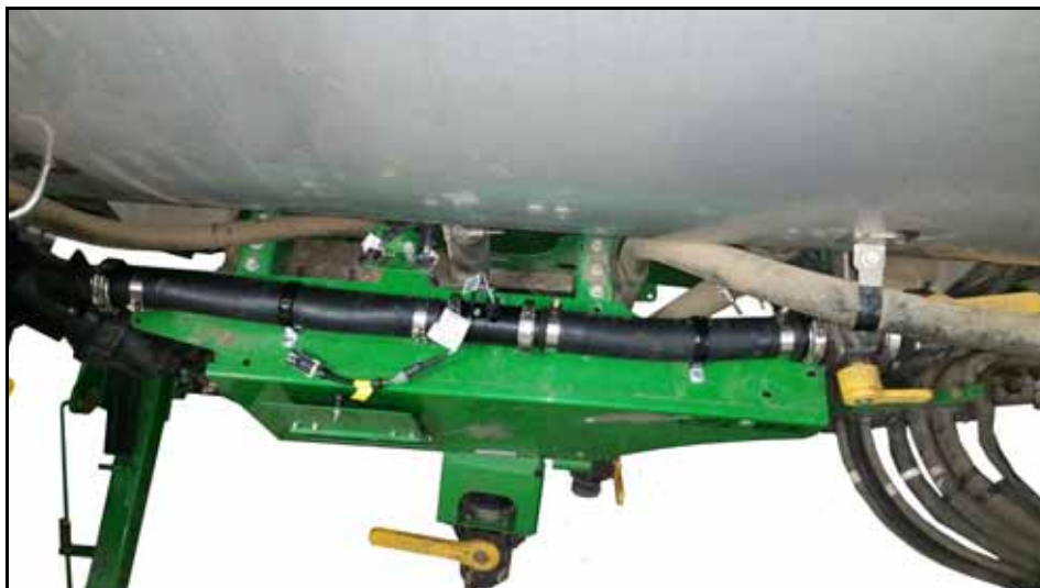
FIGURE 7. Installed Hose Clamps
