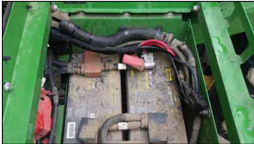
FIGURE 3. Chassis and Power Cables Connected to Battery
