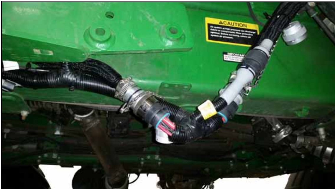
FIGURE 1. Injection Extension Cable Installation
