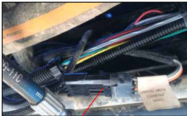
FIGURE 9. Installed Boost Box
