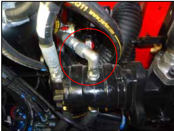
FIGURE 7. Pressure Hose Installed
