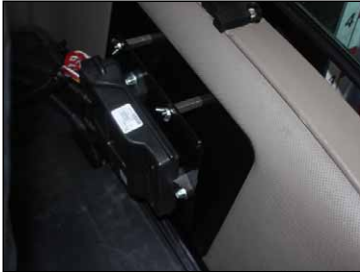
FIGURE 6. Node Cable Installed on Node
