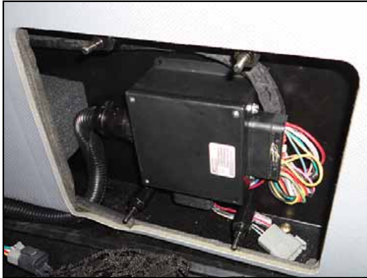
FIGURE 2. Case IH Interface Box Installed
