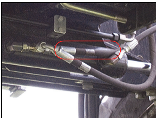
FIGURE 8. Left Steering Hose Installed
