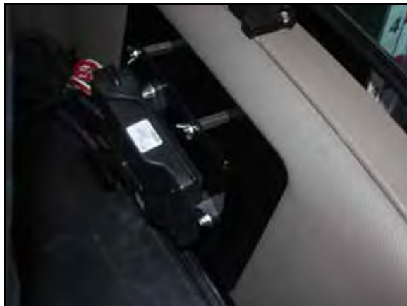
FIGURE 5. Node Cable Installed on Node
