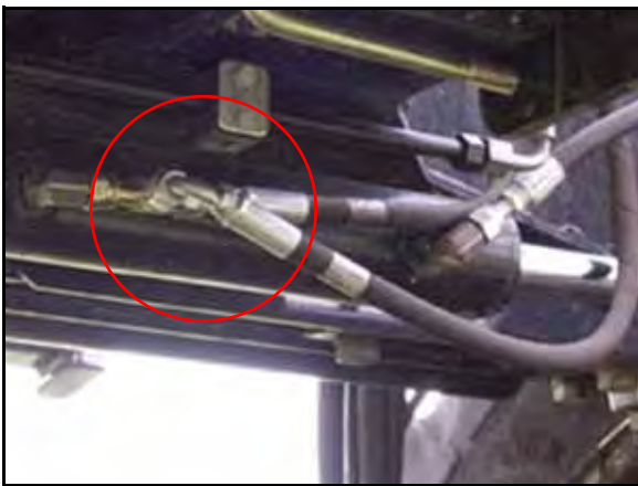
FIGURE 8. Installed Left Steering Hose
