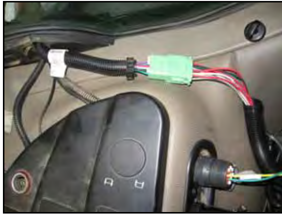
FIGURE 9. Valve Cable Routed Through Access Point
