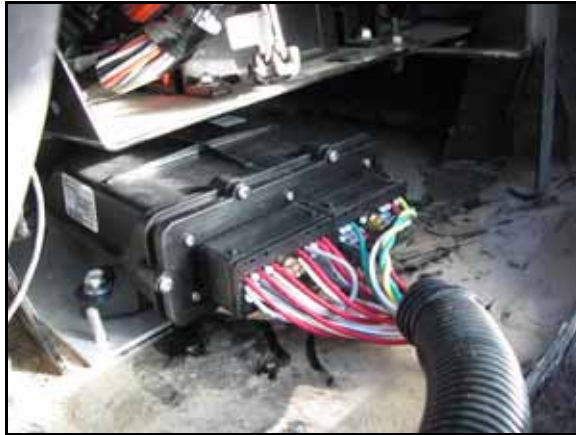
FIGURE 5. Node Cable Installed on Node
