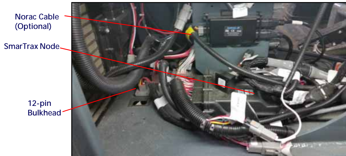
FIGURE 6. Existing Bulkhead Connection
