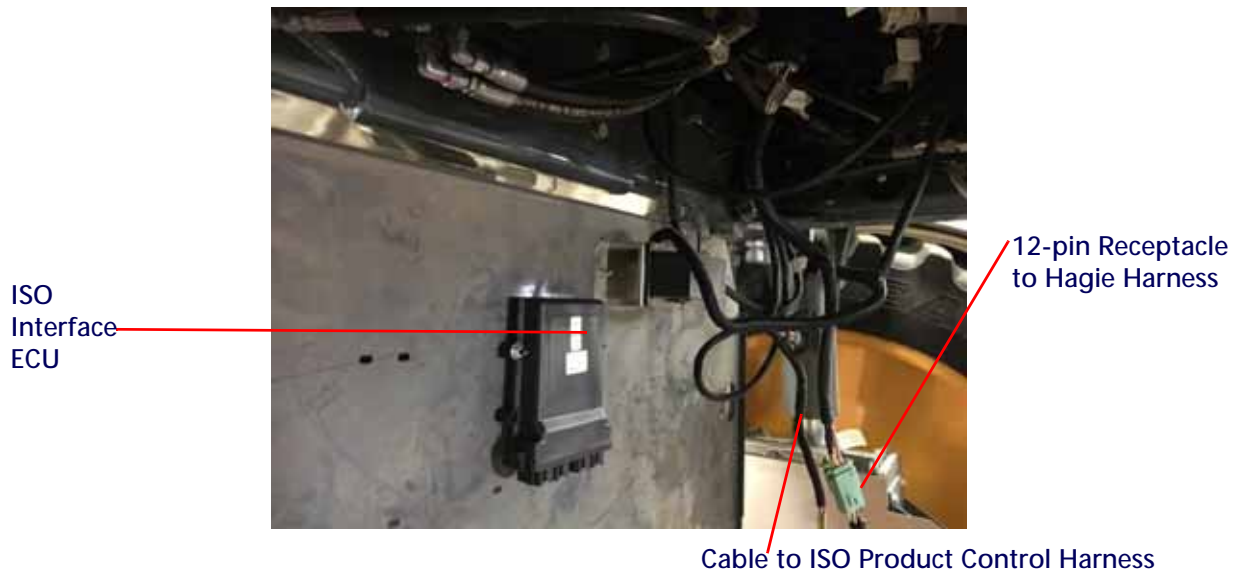
FIGURE 12. Installed ISO Interface ECU
