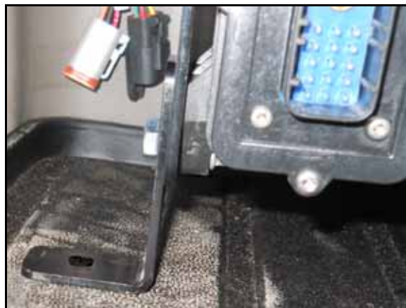
FIGURE 15. Node Support Bracket Secured to Cab Floor
