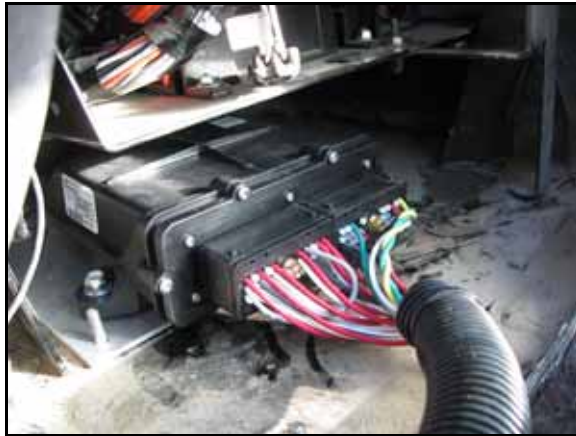
FIGURE 5. Node Harness Installed on Node
