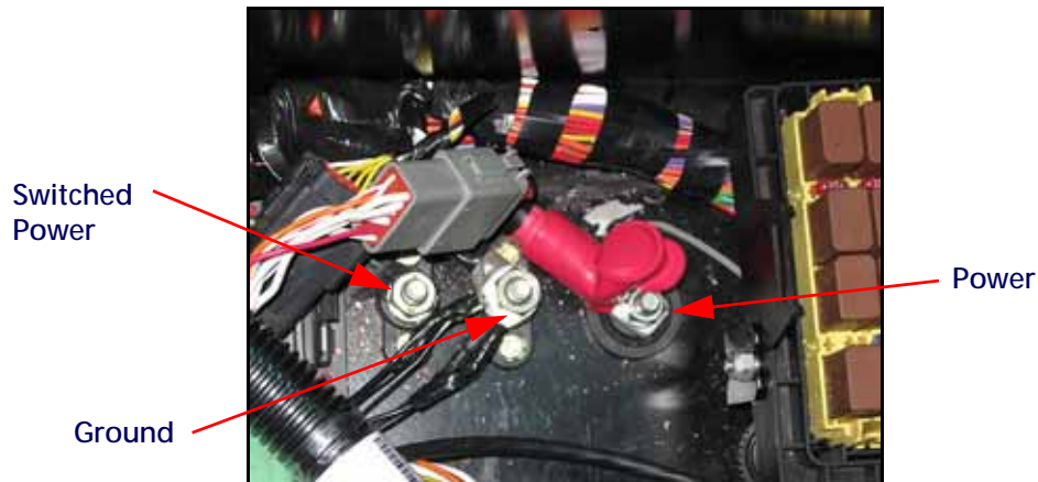
FIGURE 8. Node Harness Connected to Power Leads
