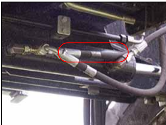
FIGURE 7. Left Steering Hose Installed
