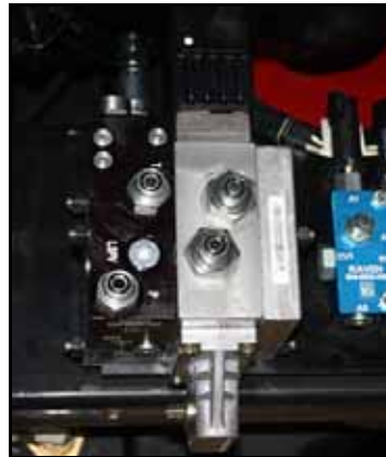
FIGURE 5. SmarTrax Valve and Flow Switch Installed
