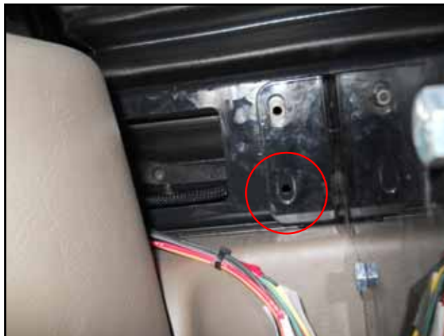
FIGURE 11. Hole Drilled in Machine's Bracket
