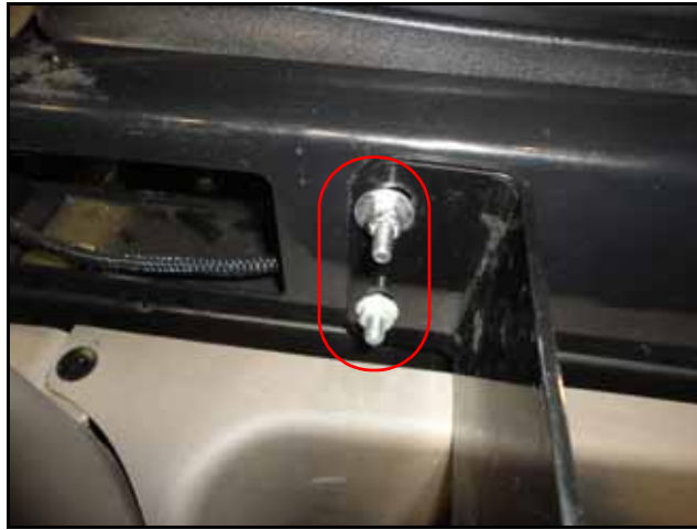
FIGURE 12. Node Mounting Bracket Installed
