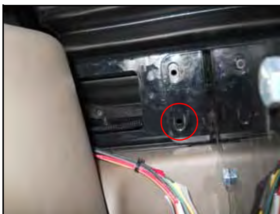
FIGURE 11. Hole Drilled in Machine's Bracket
