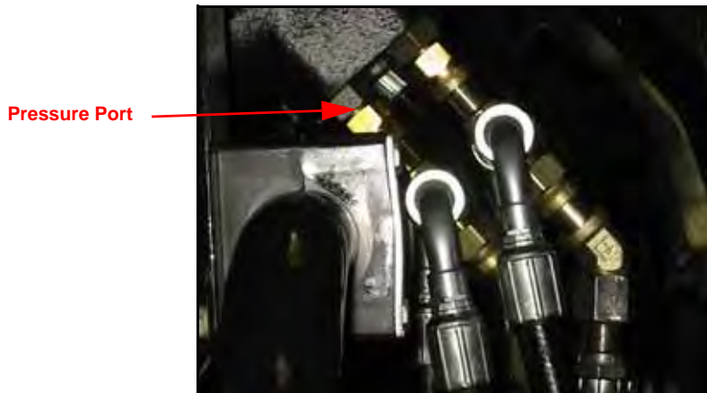
FIGURE 8. Pressure Hose Installed
