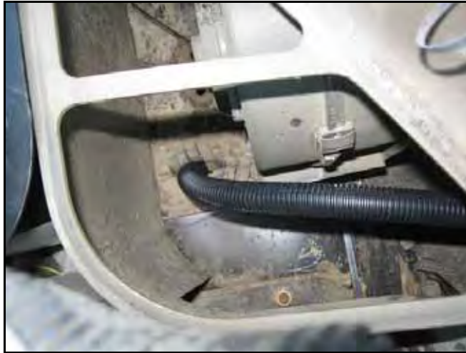
FIGURE 20. Valve Cable Routed Through Access Point
