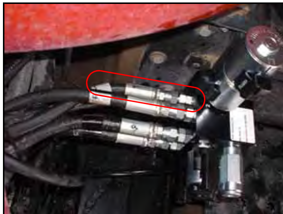
FIGURE 11. Tank Hose Installed on SmarTrax Valve
