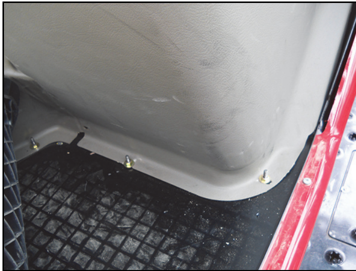
FIGURE 2. Floor Mat Removed from Cab
