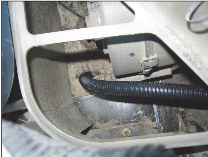
FIGURE 13. Valve Cable Routed Through Access Point
