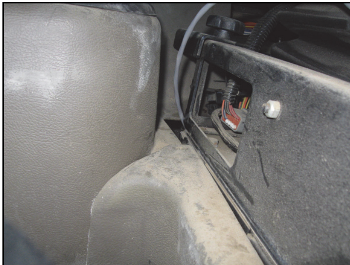
FIGURE 10. DGPS OUT Connector Routed Under Operator's Seat
