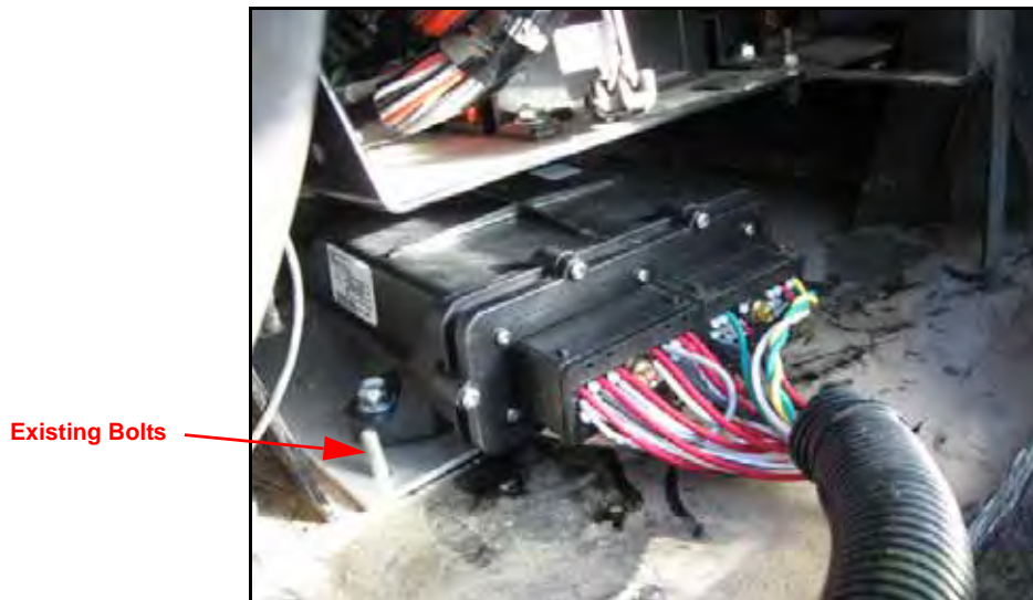
FIGURE 5. Node Mounted to Cab Floor
