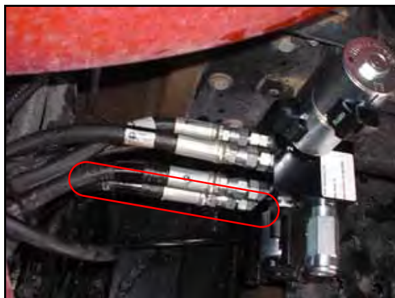
FIGURE 7. Right Steering Hose Installed on SmarTrax Valve
