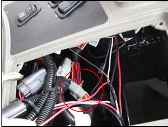
FIGURE 8. CANbus Cable Installed on Machine's CAN Connection
