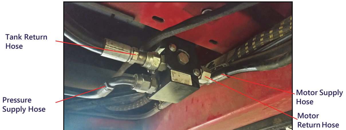
FIGURE 7. Installed PWM Valve
