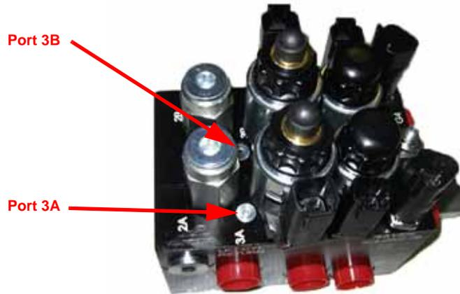
2. Locate the solenoids near ports 3A and 3B. Unscrew the large, black caps and remove the coils to make the orifice fittings more accessible.
