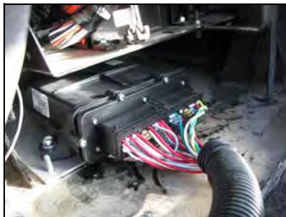
FIGURE 7. Node Cable Installed on Node
