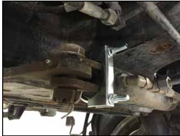
FIGURE 2. Muffler Clamp Installed on Steering Cylinder
