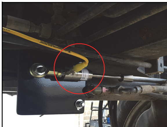
FIGURE 8. WAS Connection Installed on WAS
