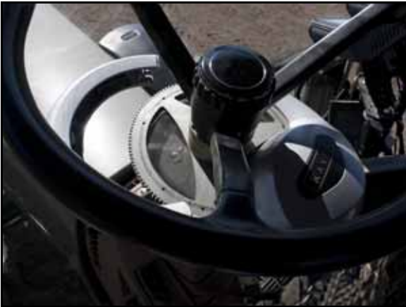
FIGURE 17. Mechanical Drive Installed
