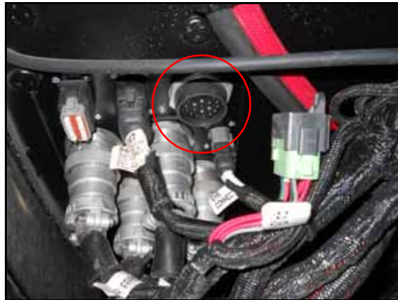
FIGURE 7. Node Harness Secured to Bulkhead
