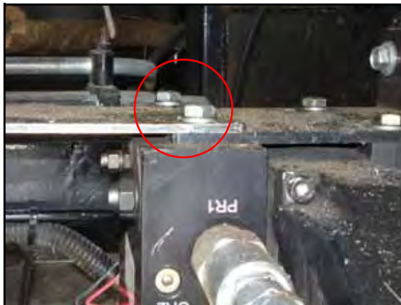
FIGURE 5. Dual POCI Valve Mounting Bracket Installed
