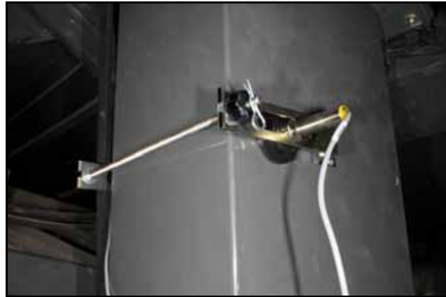
Completed Bracket Assembly
