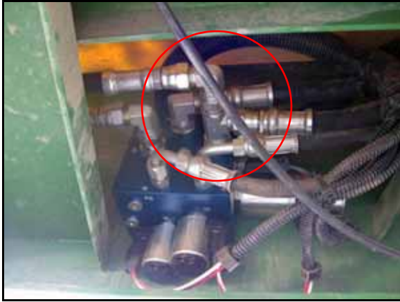
FIGURE 3. Tank Hose Installed
