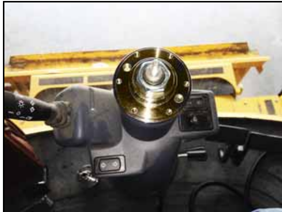
FIGURE 13. Machine's Steering Wheel Nut Installed
