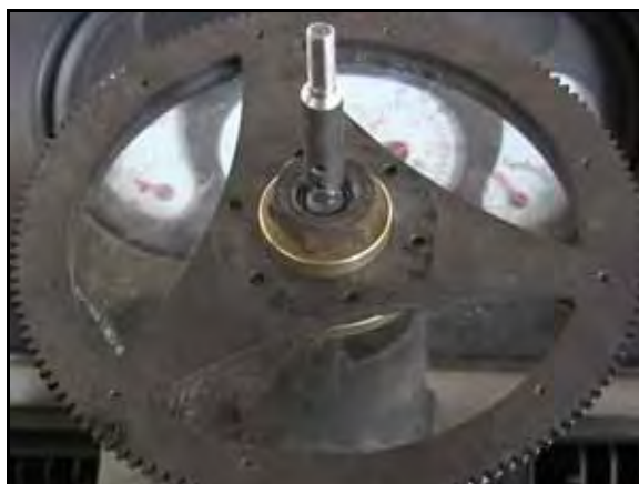
FIGURE 9. Ring Gear Assembly Installed
