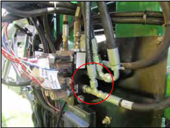
FIGURE 3. Tank Hoses Installed
