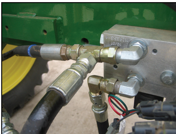
FIGURE 5. Pressure and Tank Hoses Installed
