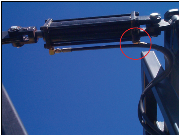
FIGURE 7. Down Hoses Installed
