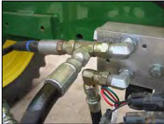
FIGURE 11. Pressure and Tank Hoses Installed
