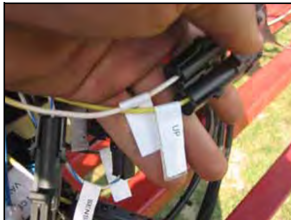
FIGURE 11. Machine's Up Cylinder Wiring
