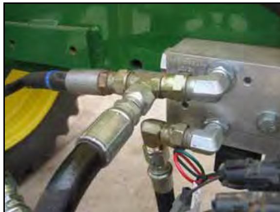
FIGURE 5. Pressure and Tank Hoses Installed
