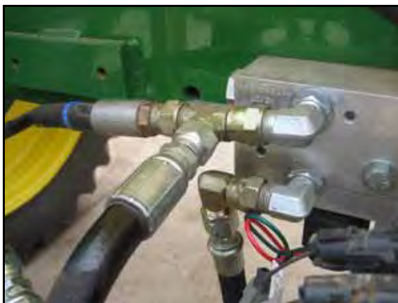
FIGURE 5. Pressure and Tank Hoses Installed
