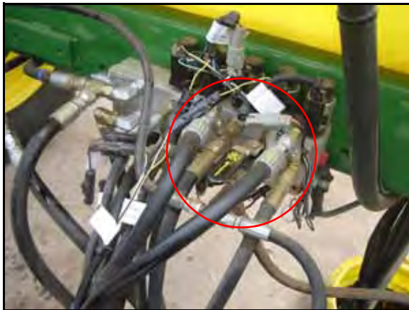
FIGURE 6. Left and Right Cylinder Hoses Installed
