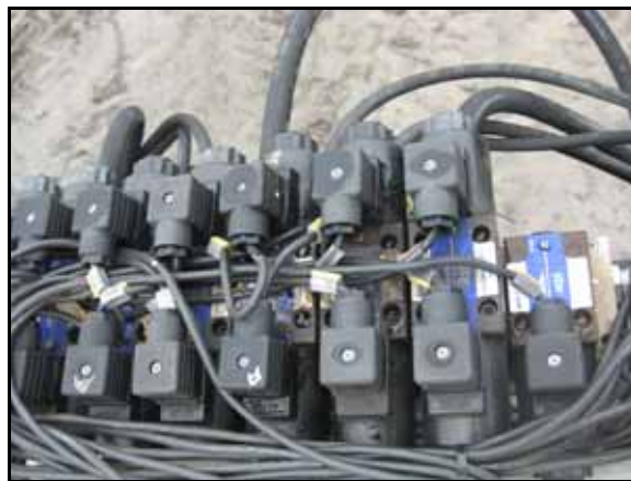
FIGURE 2. Boom Sense Adapter Cables Installed
