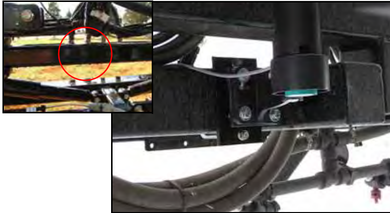
FIGURE 4. Center Sensor Installed on Machine's Center Rack
