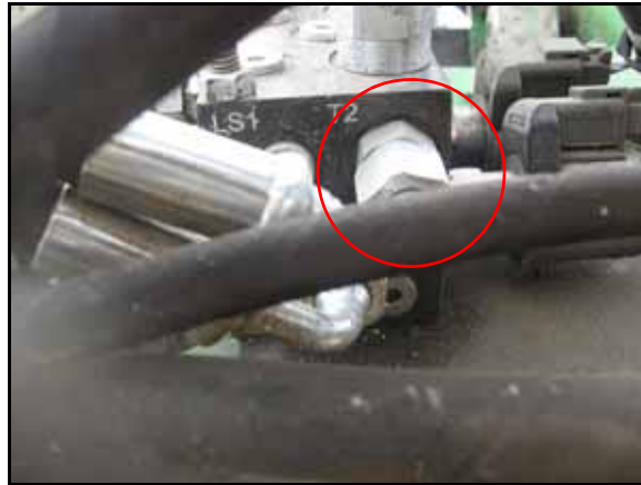
FIGURE 14. Pressure and Tank Hoses Installed on the Machine
