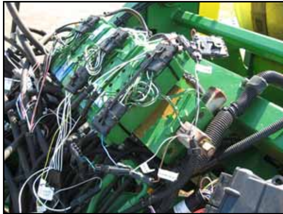
FIGURE 4. Machine's Center Rack Coils
