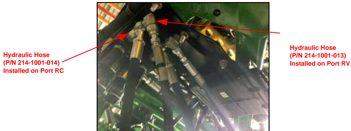
FIGURE 11. Hydraulic Hoses Installed on AutoBoom Valve
