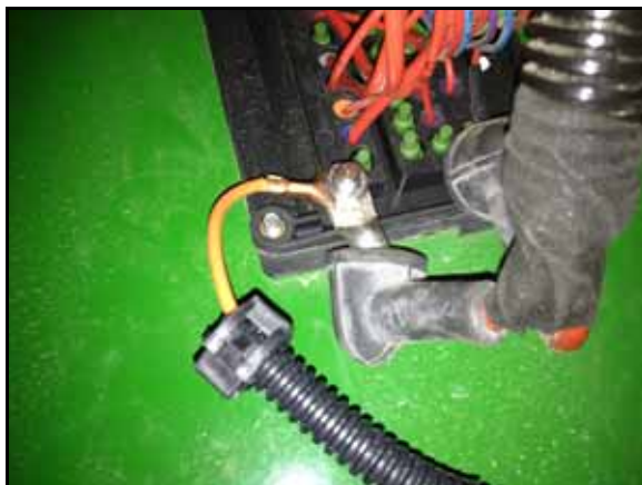
FIGURE 5. Power Cable Installed on Switched Power Post
