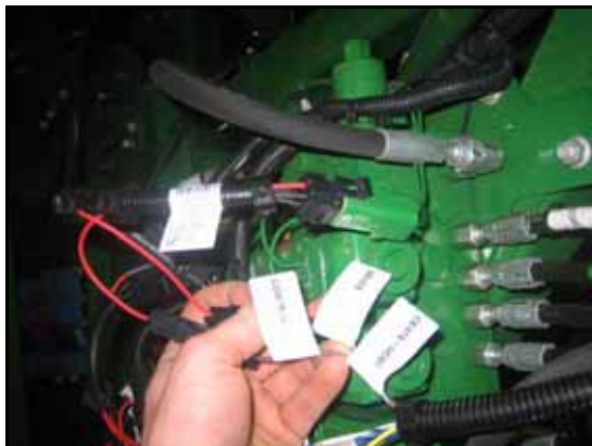
FIGURE 12. Machine's Center Boom Function Coils
