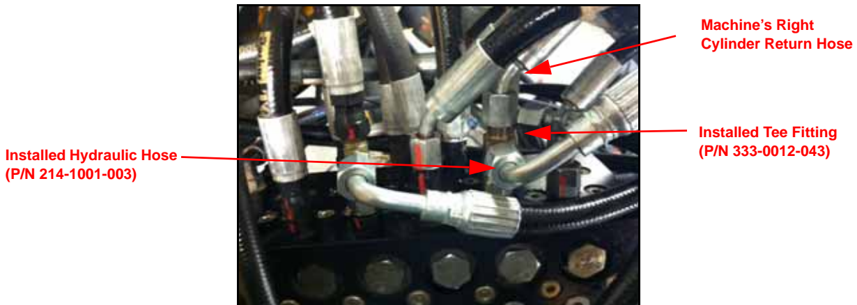
FIGURE 11. Tee Fitting Installed in Machine's Right Cylinder Return Port
