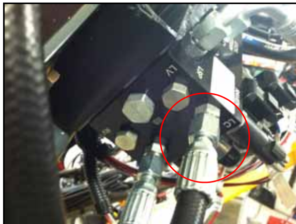
FIGURE 6. Left Cylinder Hose Installed on AutoBoom Valve
