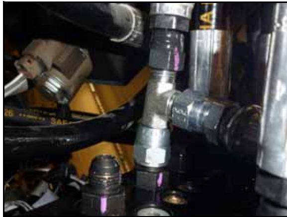
FIGURE 5. Left Cylinder Hose Installed Machine's Hydraulic Valve
