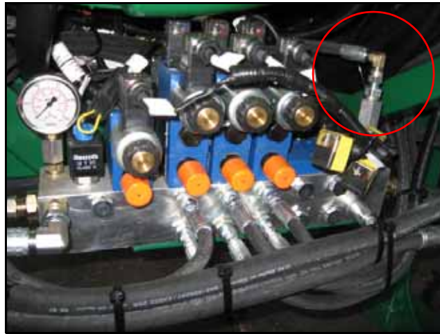
FIGURE 11. Load Sense Hose Installed on the Machine's Hydraulic Valve
