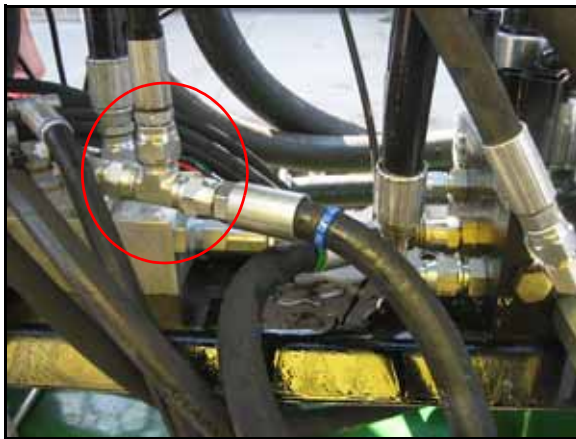
FIGURE 12. Tank (Return) Hose Installed
