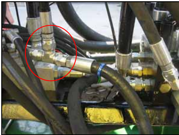
FIGURE 6. Tank (Return) Hose Installed
