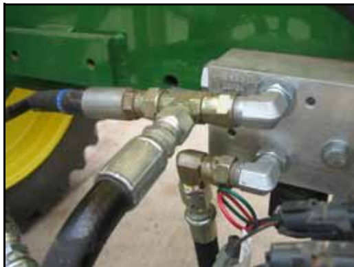
FIGURE 10. Pressure and Tank Hoses Installed
