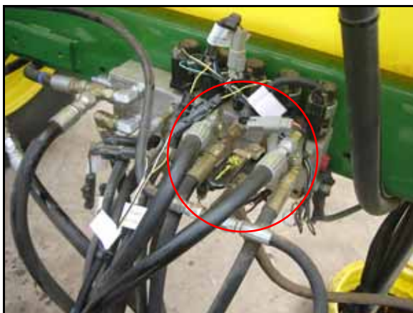
FIGURE 5. Cylinder Hoses Installed
