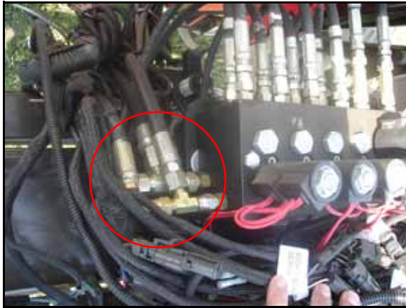
FIGURE 3. Pressure and Tank Hoses Installed
