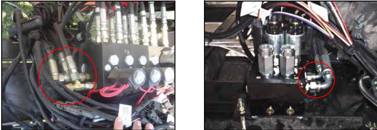
FIGURE 9. Pressure and Tank Hoses Installed
