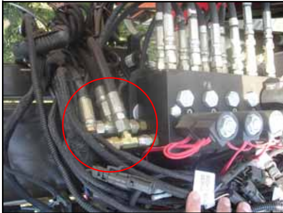
FIGURE 3. Pressure and Tank Hoses Installed
