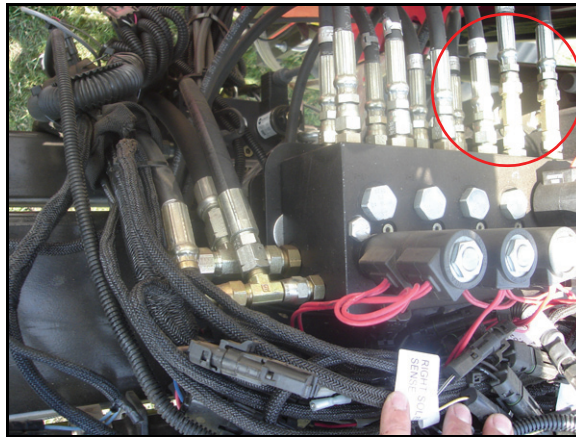
FIGURE 4. Cylinder Hoses Installed on Machine's Hydraulic Valve
