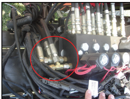
FIGURE 3. Pressure and Tank Hoses Installed
