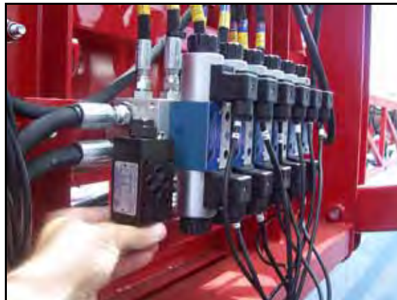
FIGURE 9. Sub-plate Lockout Valve Installed
