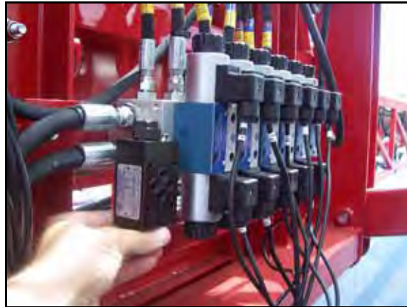
FIGURE 6. Sub-plate Lockout Valve Installed
