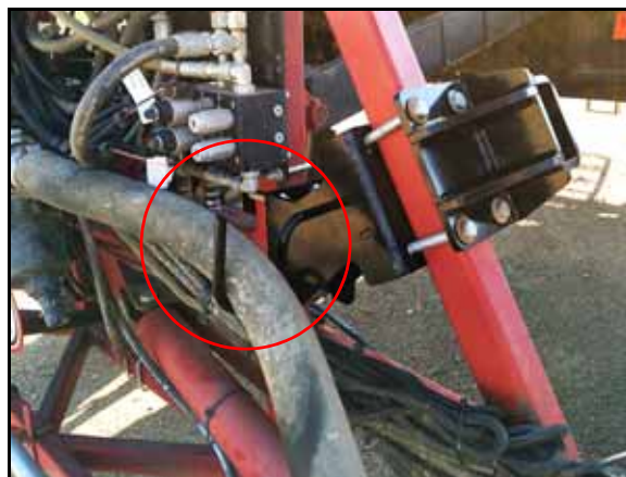
FIGURE 14. Hose Retainer Bracket Installed
