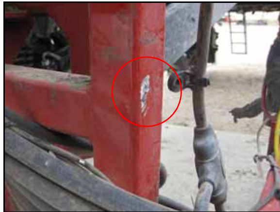
FIGURE 11. Stud Removed from Machine's Frame
