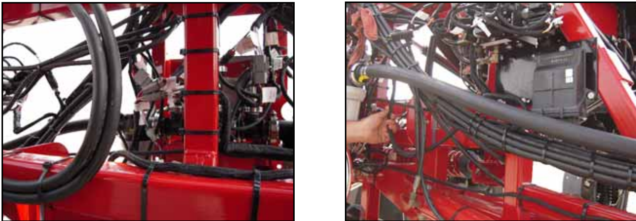
FIGURE 5. AutoBoom Harness Cable Installed
