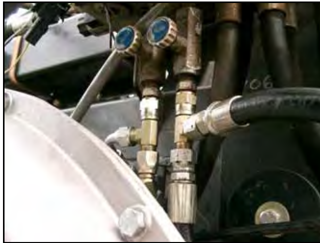
FIGURE 10. Left and Right Cylinder Hoses Installed
