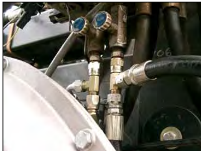
FIGURE 4. Left and Right Cylinder Hoses Installed
