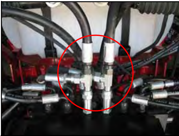
FIGURE 4. Left and Right Cylinder Hoses Installed
